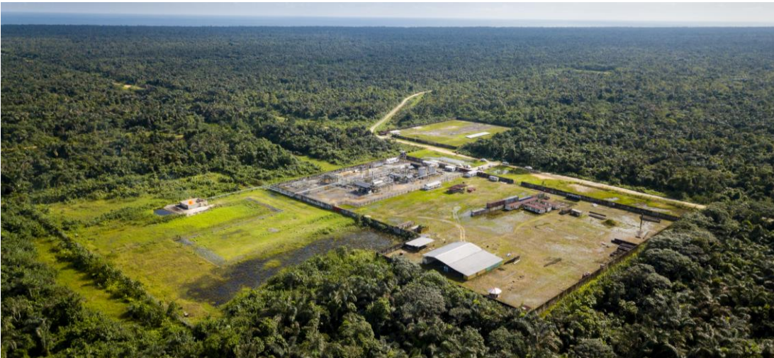
Stubb Creek oil production facility
