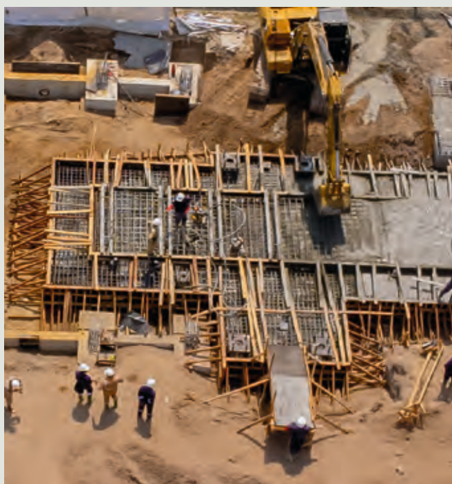
Compression project shallow foundations works, Savannah's Uquo CPF, Nigeria
