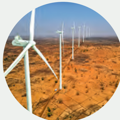
A visual representation of Savannah's proposed Parc Eolien de la Tarka wind farm project, Niger
