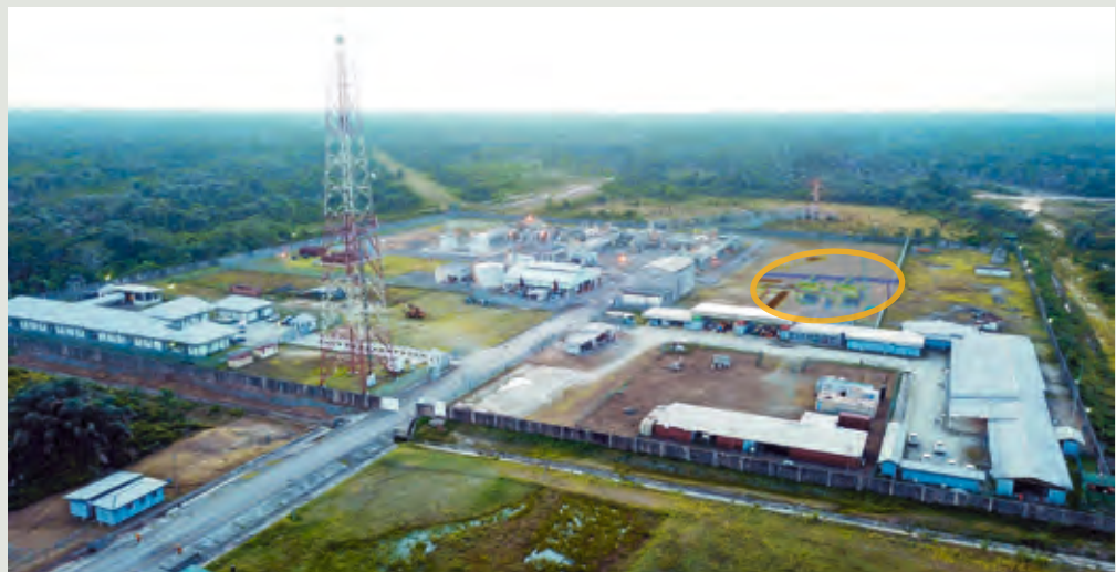
Current view of Savannah's Uquo CPF, Nigeria (Ellipse indicates the new compression system location)
