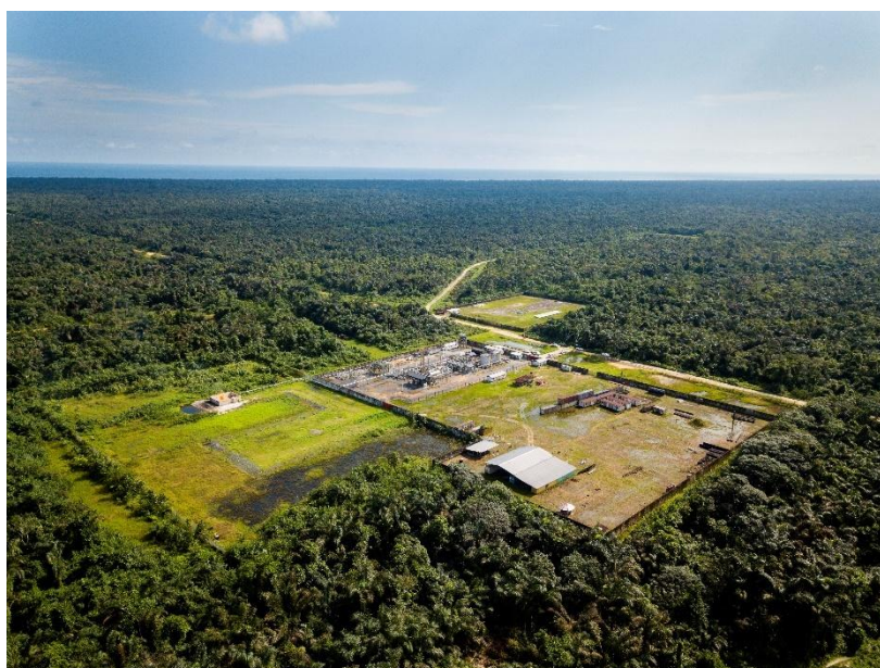
Savannah's Stubb Creek Field, Oil Processing Facility, Nigeria
